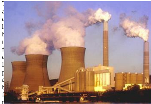
Pittsburgh's Bruce Mansfield coal-fired power plant northwest of Pittsburgh, Pennsylvania (Photo by Kiyu Komoda)
